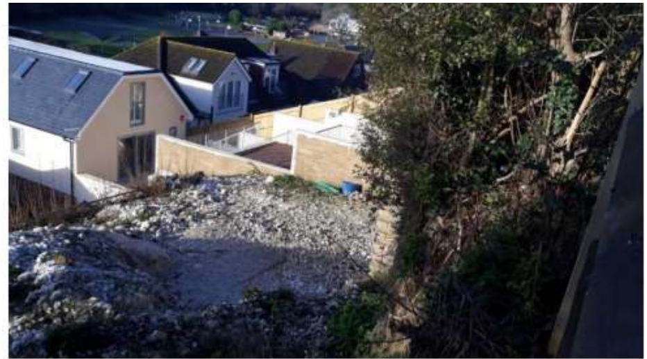
VIEW WEST FROM UPPER LEVEL OF SITE
