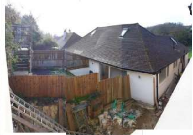
REAR OF EXISTING BUNGALOWS
